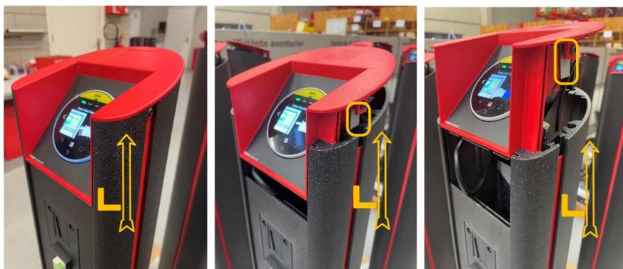
3. The top can now be lifted out of the pillar, only the cable is still connected to the Nayax module.
